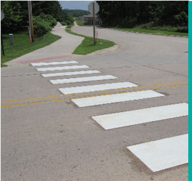
Figure 10. A highly visible, clearly marked pedestrian crosswalk (Image: Neal Hawkins, Center for Transportation Research)
