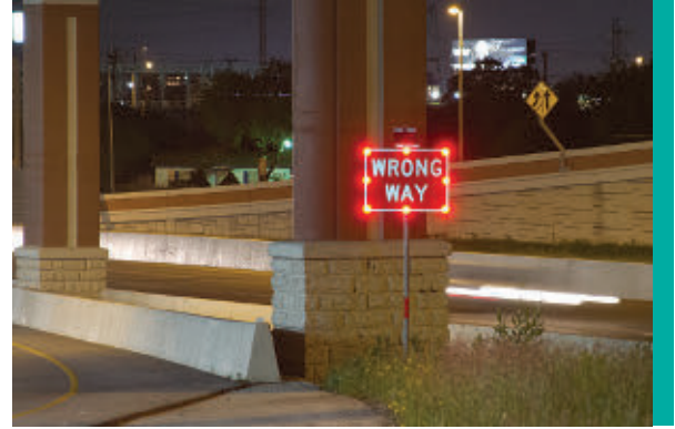
Figure 7. A Wrong Way sign with LED enhancement (Image: Traffic & Parking Control Co. Inc. (TAPCO))
