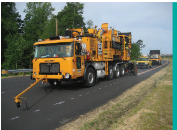
Figure 15. Yellow spray thermoplastic edge lines being applied to an interstate highway near Raleigh, N.C. (Image: ATSSA Pavement Marking Division)
