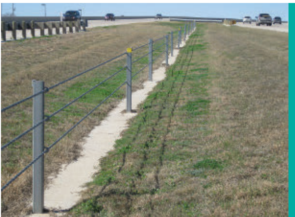
Figure 31. Installed cable median barrier (Image: Gibraltar)
