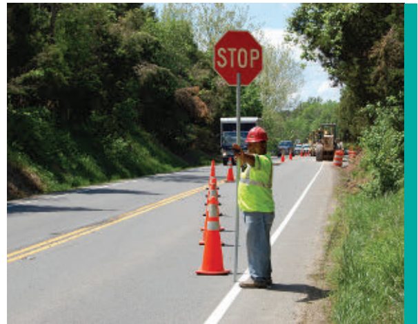
Figure 30. A road worker in a retroreflective vest and hard hat, Manassas, Va. (Image: James Scott Baron, ATSSA)
