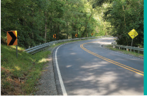
Figure 6. Post-mounted chevrons in a curve, Route 218, King George County, Va. The school-area sign (right) warns of pedestrians in the area (Image: James Scott Baron, ATSSA)
