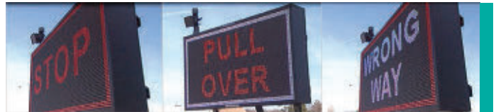
Figure 28. Wrong-Way Entry ITS Warning System on the New York Thruway (Images: New York State Media Services Center)
