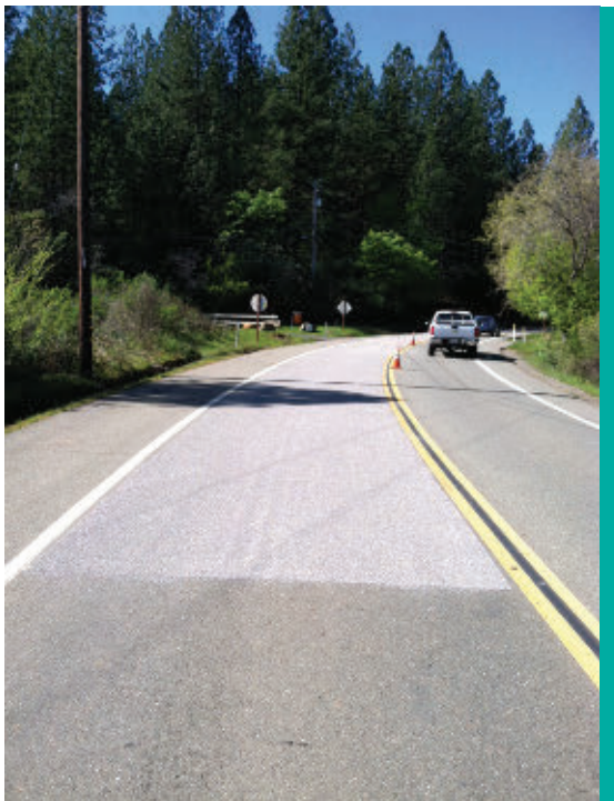
Figure 18. HFST in Placer County, Calif. (Image: Richard J. Baker, DBI Services)
