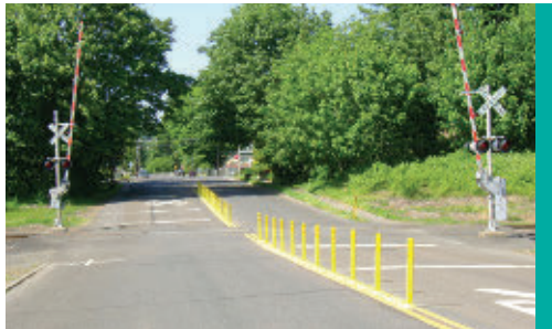
Figure 21. Flexible channelizing posts at a railroad crossing, Washougal, Wash. (Image: Pexco LLC)
