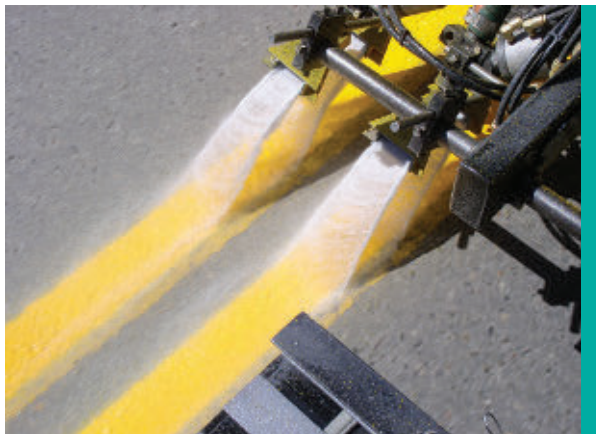
Figure 16. Glass beads being applied during a double-yellow-centerline plural-component epoxy application (Image: ATSSA Pavement Marking Division)
