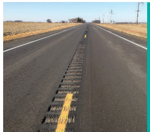
Figure 3. A sample of milled centerline rumble strips (Image: Neal Hawkins, Center for Transportation Research)
