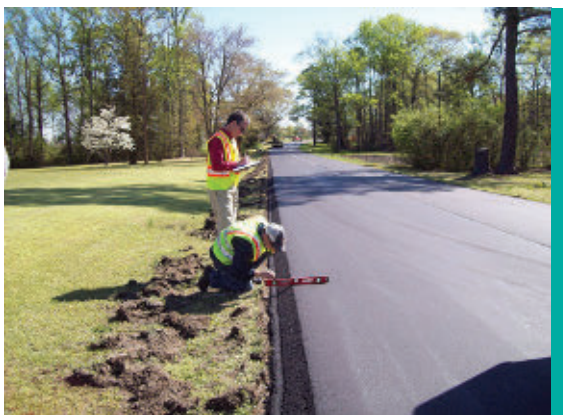
Figure 19. Federal Highway Administration's (FHWA's) Andy Mergenmeier and Chris Wagner gathering data on a new Safety Edge SM project (Image: Frank Julian, FHWA)
