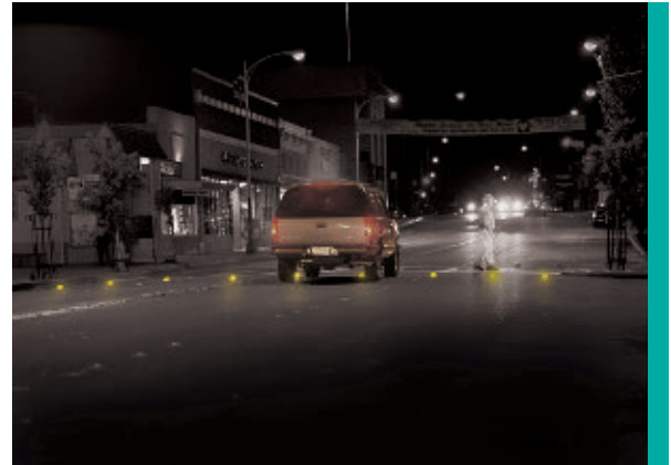
Figure 11. In-pavement lighting improves the visibility of the crosswalk at night (Image: LightGuard Systems Inc.)
