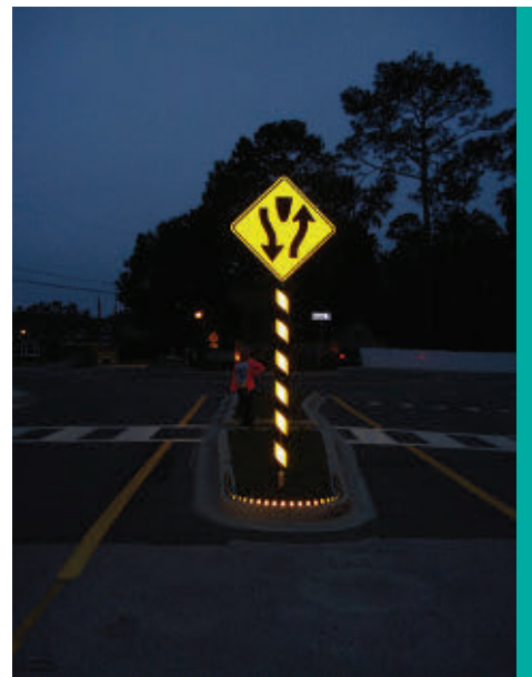
Figure 26. Reflective material on the concrete curb below the sign and its post alerts motorists there is a curb on the roadway (Image: Professional Pavement Products, Inc.)
