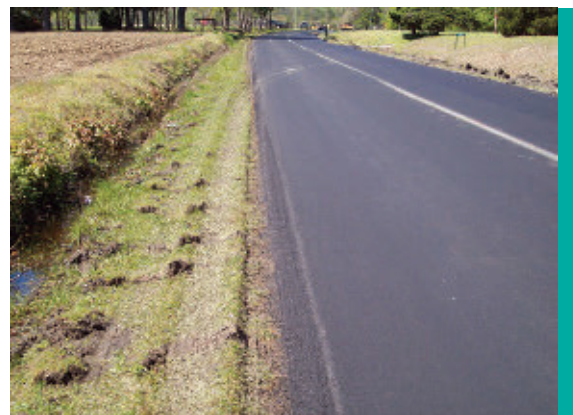
Figure 20. Note the tire tracks on the shoulder and onto the roadway. The edge of the Safety Edge SM remained unharmed after being crossed by a fully loaded asphalt truck during road construction (Image: Frank Julian, FHWA)
