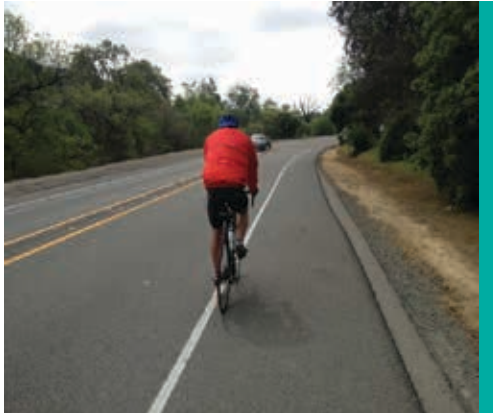
Figure 29. Sample of Wider Shoulder (Image: Caltrans)
