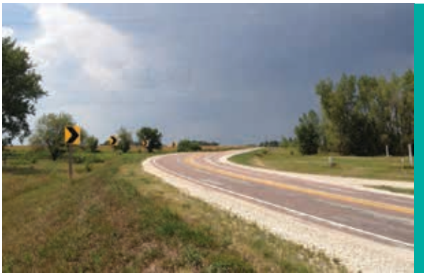
Figure 3. Sample of Installed Chevron (Image: Neal Hawkins)
