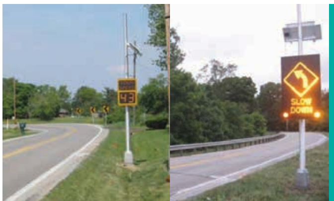
Figure 4. Two Examples of Installed DCWS (MTC 2009)
