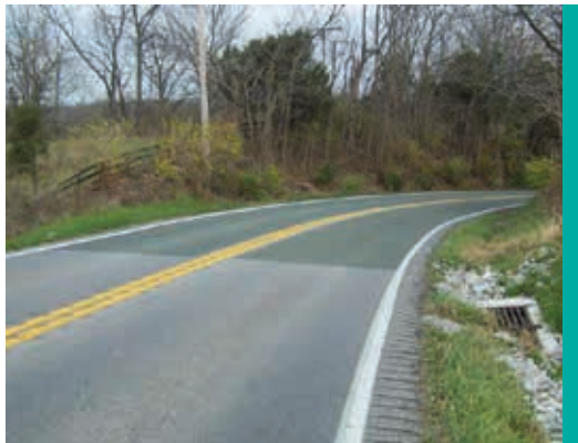
Figure 8. Sample of High-Friction Surfacing Treatment on a Roadway, Madison County, Ky. (Image: Kentucky Transportation Cabinet)
