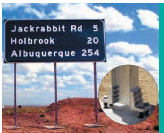
Figure 24. An Information Sign with Breakaway Supports (FHWA 2012f)
