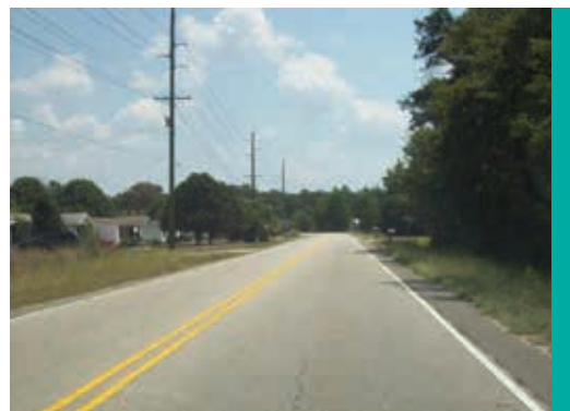
Figure 32. Site 3: Driving East on State Route 2220 (NCDOT 2014)
