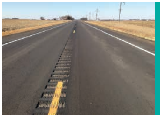
Figure 15. Sample of Installed Milled CLRS (Image: Neal Hawkins)
