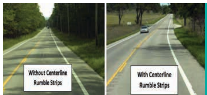
Figure 16. Before (left) and after (right) Pictures of the CLRS Installation (Datta et al. 2012)
