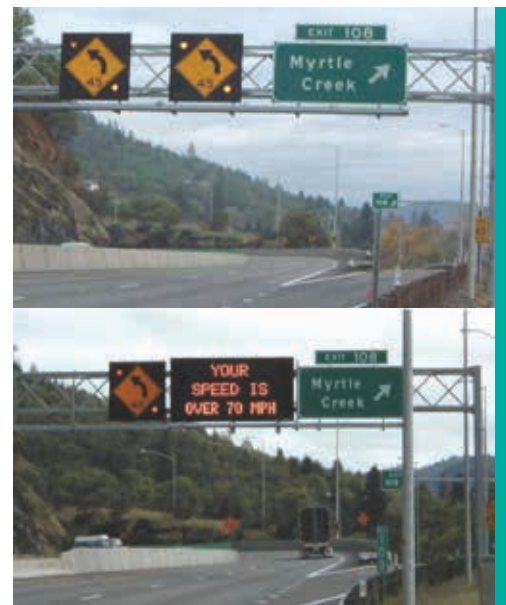
Figure 5. Before (top) and after (bottom) Pictures of DCWS at Interstate 5 (Bertini et al. 2006)
