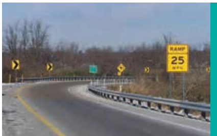
Figure 6. Example of Advisory Ramp Speed Sign and Chevrons (FHWA 2009b)
